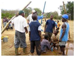
MANUAL DRILLING WITH THE SO CALLED SHIPO METHOD
