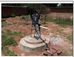
An improved well with a well slab and a low cost hand pump.
