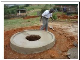
Improving an open hand dug well with a well slab.
