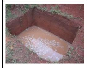
Photo 3. When it rains the pit fills up and water is infiltrating in the ground
