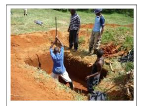
Photo 1. A recharge hole is made with a Soil punch. This hole passes the compact clay layer and in this case is 5 meters deep
