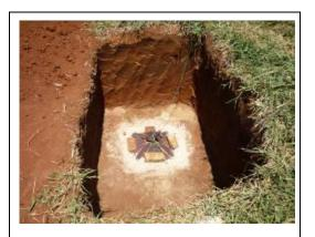
Photo 2. The hole is filled with gravel and covered by a sand filter that is then covered with a cloth filter. A rope is attached to the cloth filter to pull it up for cleaning
