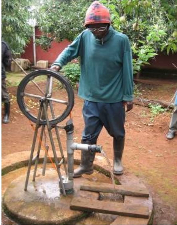
7 A Tube recharge system installed at a family in Njombe in Tanzania in 2011
