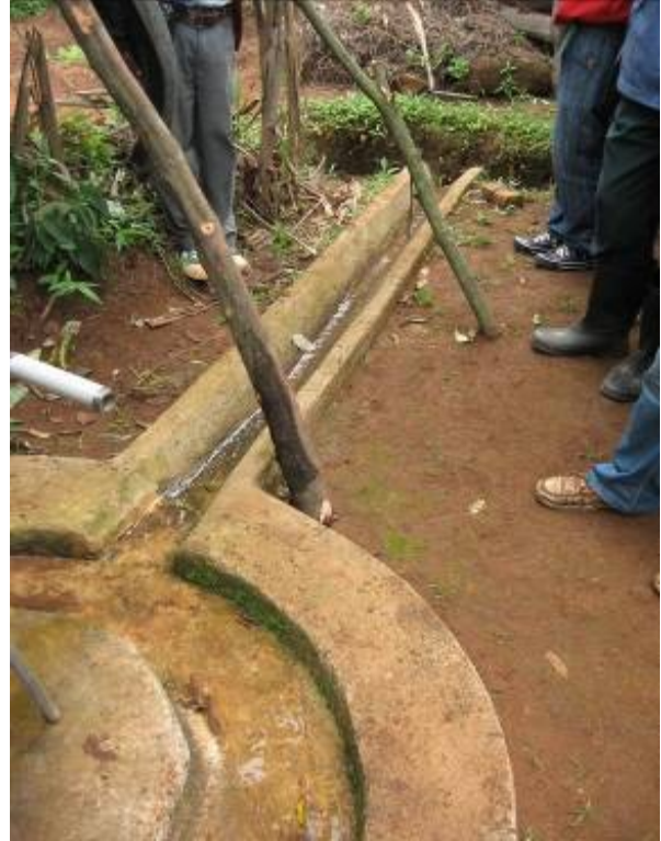
8 The water from the roof and run off water from the area around the house is led to the pit.
