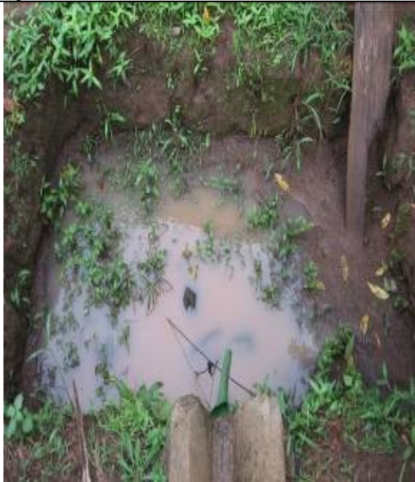
9 Each rain the pit fills up and water infiltrates in the ground via a cloth filter and a sand filter
