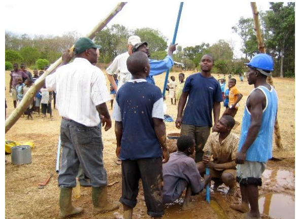
Manual Drilling with SHIPO method. A well can be drilled for a cost of $200 - $1500/well. The price depends on the local geology.
