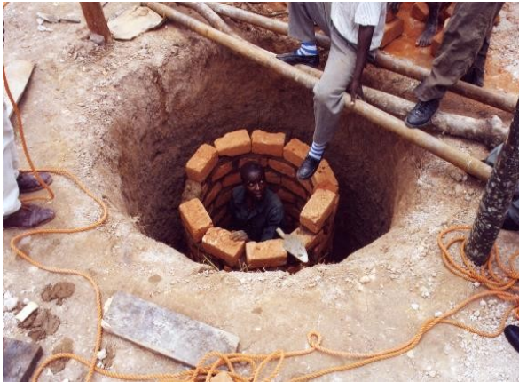
Lining hand dug wells to avoid collapsing
