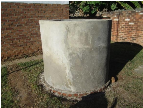
Wire cement water tank. Constructed from baked bricks, cement and galvanized wire. Can be used for rainwater harvesting or to store water from (hand)pumps. Cost of a tank of 2000 liters is $40 - $60.
