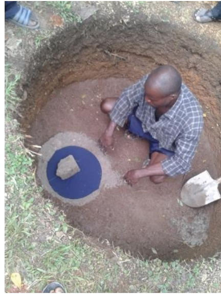
Tube recharge. A low-cost way to recharge (rain)water into the soil which can lead to higher water levels in (dry) wells.
