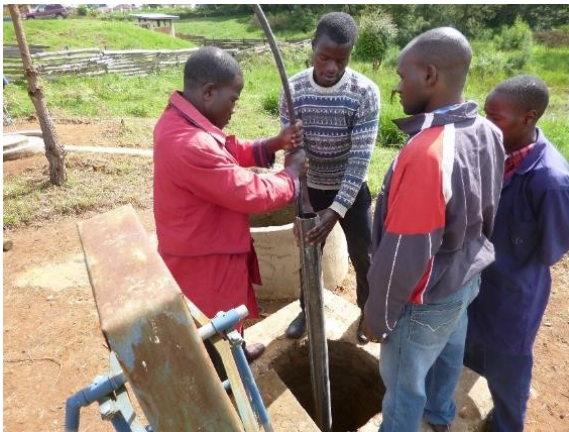
Deepening a hand dug well with the tube bailer, through inserting a filter screen at the bottom of the well. This allows wells that dry up to provide water year round.
