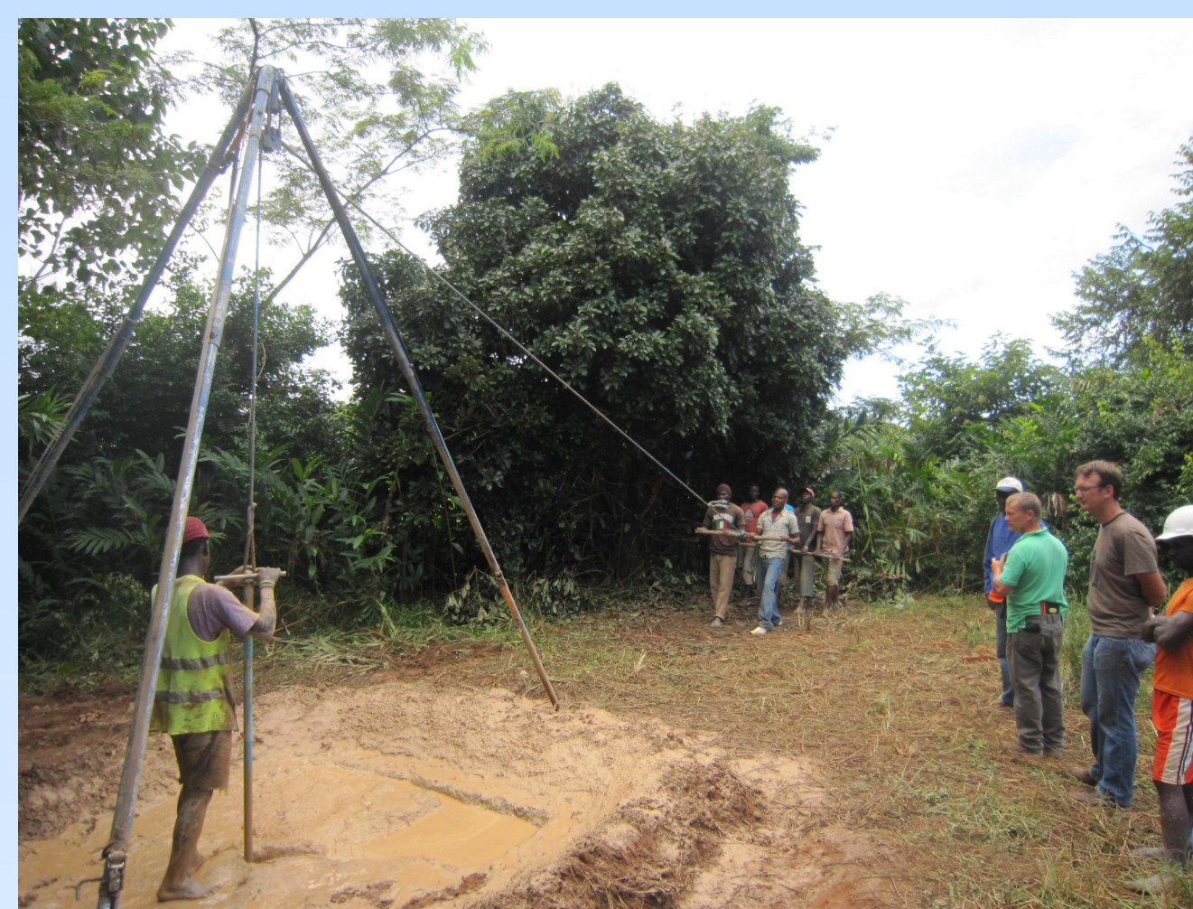
New wells can be dug or hand drilled with options. Cost of well (40 m deep) $500-$1500
