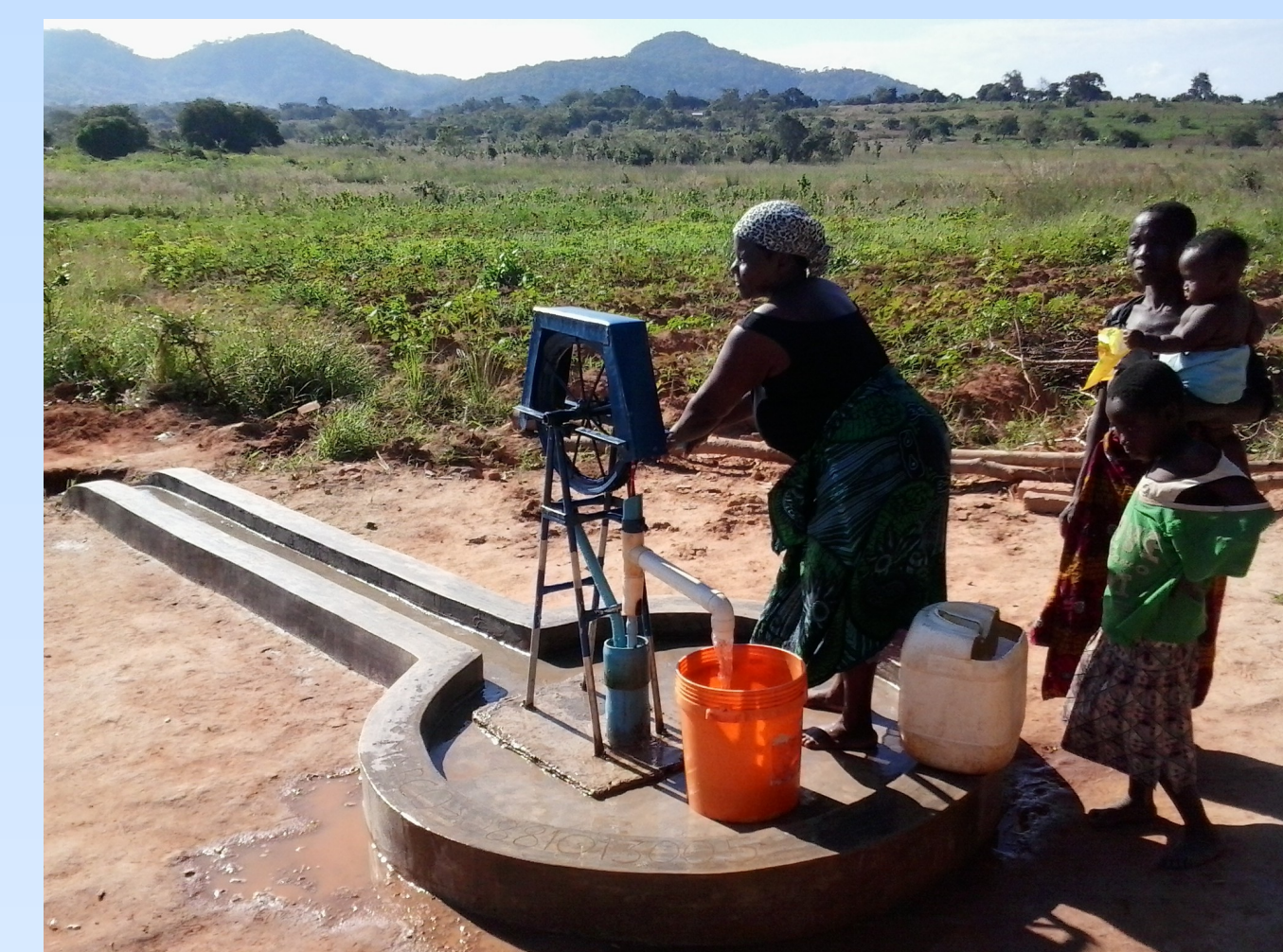
Wells can be upgraded with a well cover and a Hand pump. Cost cover and hand pump $120
