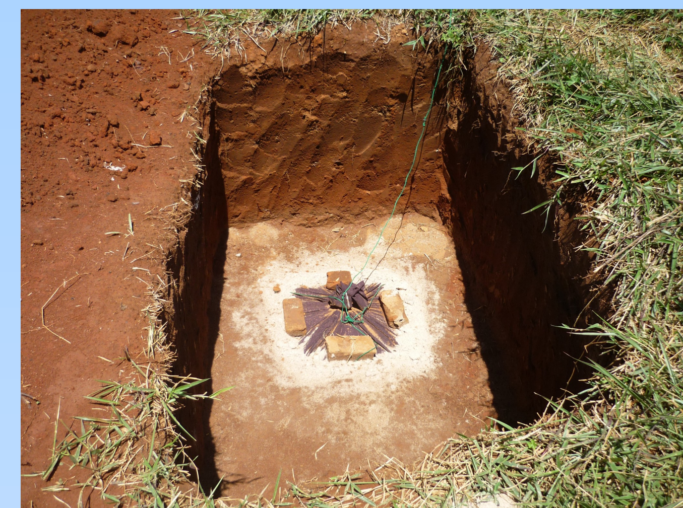
Dry wells can be restored with recharge options like a Tube re-charge , Cost materials $10
