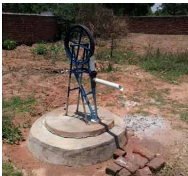
Top photo; Prefabricated well cover with bolts for mounting a rope pump.
