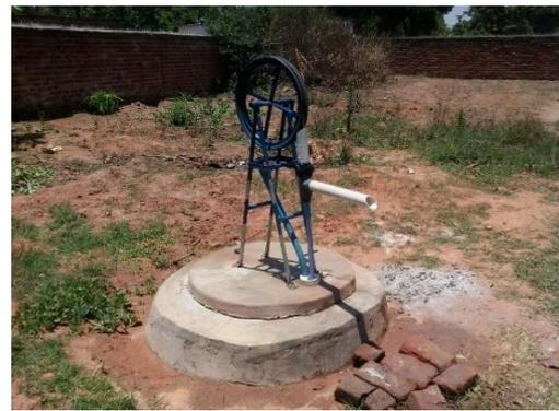
An improved well with a well slab and a low cost hand pump.
