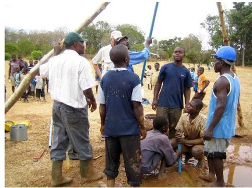
MANUAL DRILLING WITH THE SO CALLED SHIPO METHOD
