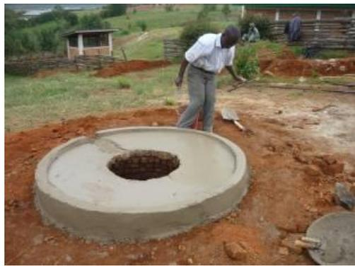
Improving an open hand dug well with a well slab.
