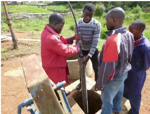
MAKING A WELL DEEPER WITH THE WELL PIPE TECHNOLOGY
