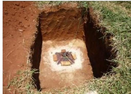
Photo 2. The hole is filled with gravel and covered by a sand filter that is then covered with a cloth filter. A rope is attached to the cloth filter to pull it up for cleaning
