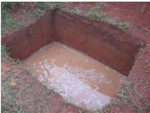
Photo 3. When it rains the pit fills up and water is infiltrating in the ground
