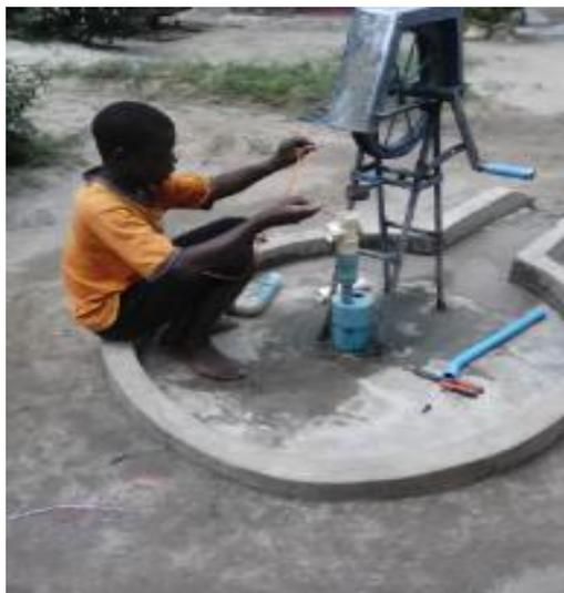
Photograph 2. Maintenance of Rope pump
