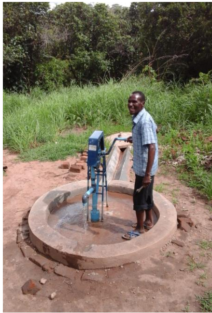
Figure 1: Communal Rope pump installed on an existing hand dug well (source: Reinier Veldman)
